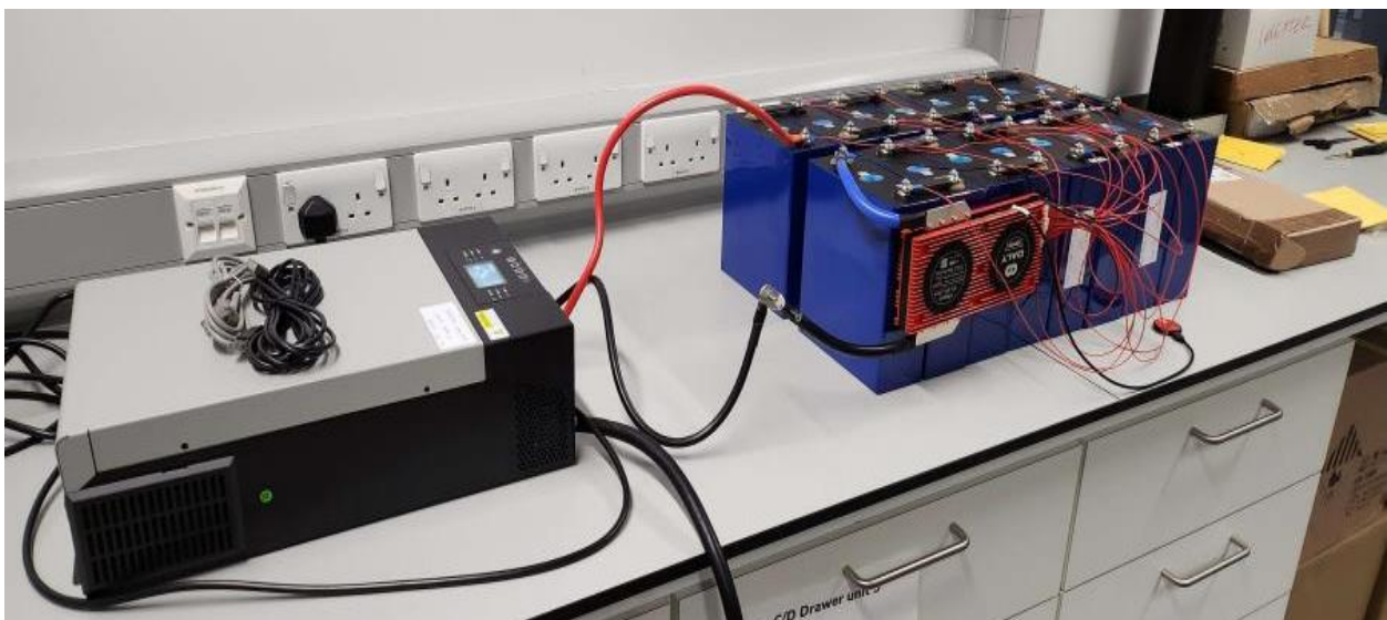
Figure 7 - Image showing testing of LiFePO 4 battery with hybrid inverter system.
